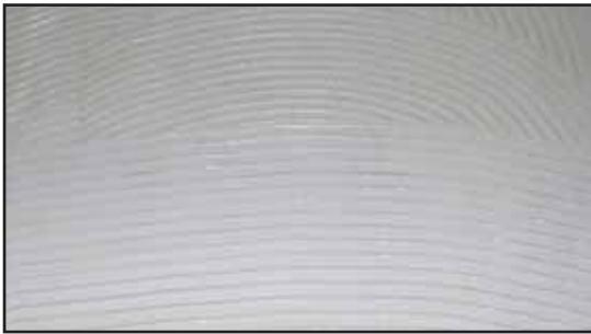
Example of properly troweled adhesive application
