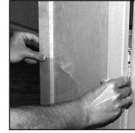
**Step 6:** Press the door firmly onto the door brackets with the two sided tape. Put pressure directly on the sides, in position with the brackets to allow for good adhesion.
