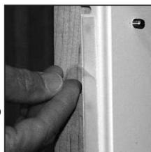
**Step 8:** Fasten the brackets to the door using the tape as a temporary hold while you insert #6 x 1/2" wood screws.
