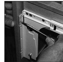
**Step 5:** Peel off the exterior layer of tape. Now carefully line up your desired door position by eyesight using the drawer above and any cabinets to your left or right as a gauge for correct alignment.
