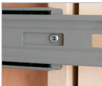
Front of slides mounts to the face frame of the cabinet
